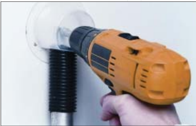
Vacuum cleaner and cowl being used for drilling
